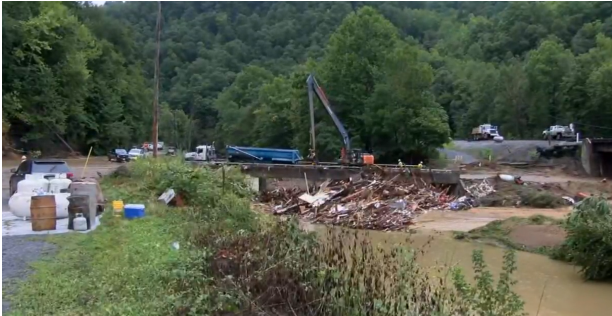
Figure 6-22: Debris collected at a bridge in Hurley, 2021 36
